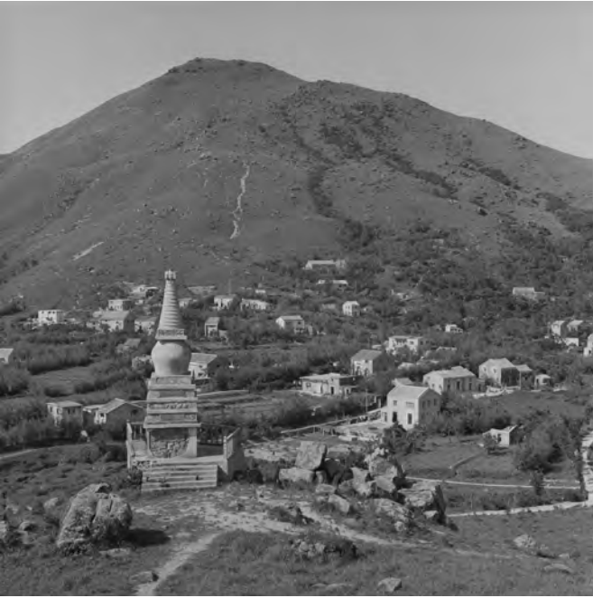
1960 年代昂坪地區佛教山林建築群，背景為彌勒山。 The Buddhist settlements in the Ngong Ping area in the 1960s, with Nei Lak Shan visible in the background.
